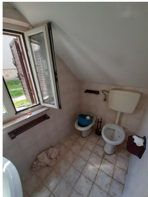
Bagno piano terra
