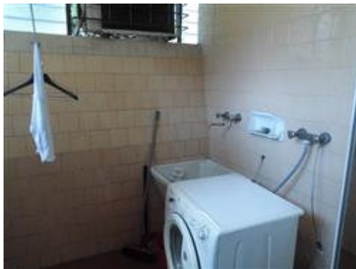
lavanderia piano interrato
