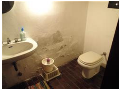
bagno piano interrato
