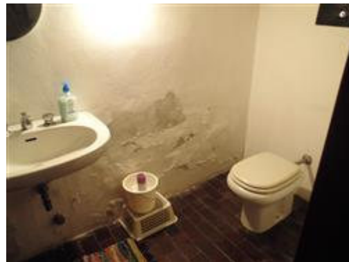
bagno piano interrato
